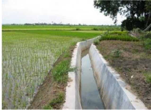
Gambar 2. Saluran Irigasi Sekunder http://theworldagriculture.blogspot.com/2013
