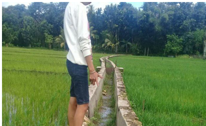
Gambar 4. Saluran Drainase di Sawah https://www.google.com/search?q=drainase+sawah&tbm
